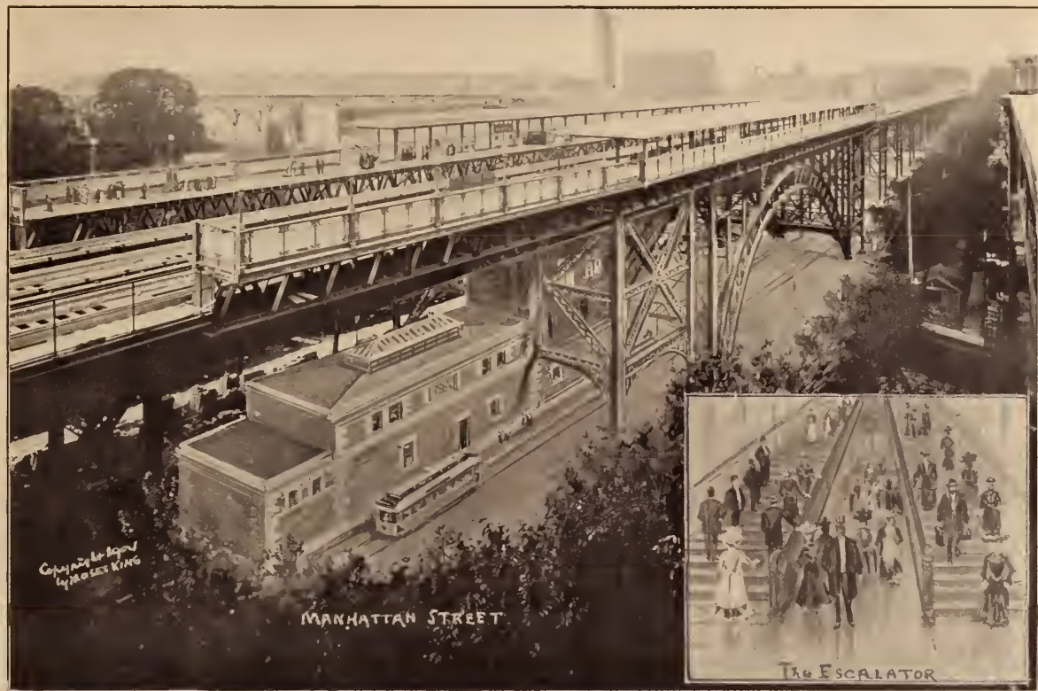
MANHATTAN VALLEY VIADUCT. FROM 123RD TO 135TH STREET. STATIONS BUILT BY HECLA IRON WORKS OF BROOKLYN. The Great Arch at Manhattan St. spans 170 ft. Tracks 50 ft. high. Otis Escalator, capacity 20,000 passengers an hour, at the Manhattan St. Station.
